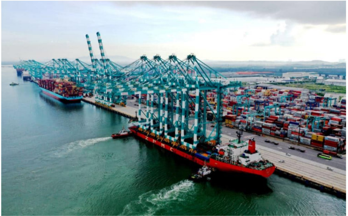
Four more STS cranes will be delivered in Q3 2020
